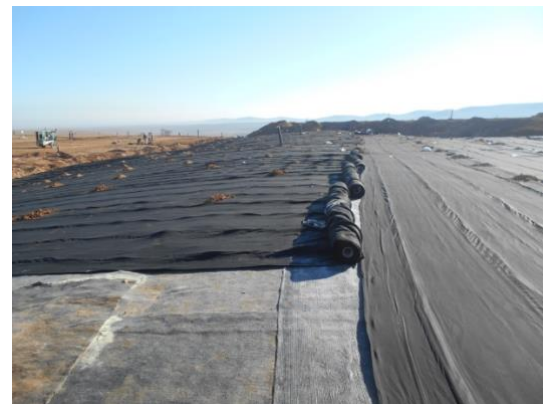
Installation of DRAINTUBE FT on the GCL
