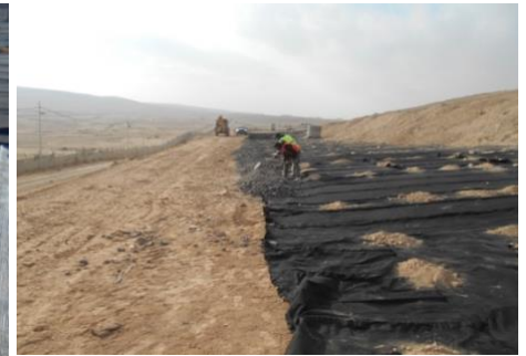
Top Soil to cover the DRAINTUBE FT
