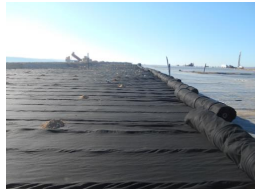
Installation of DRAINTUBE FT above GCL for surface water drainage
