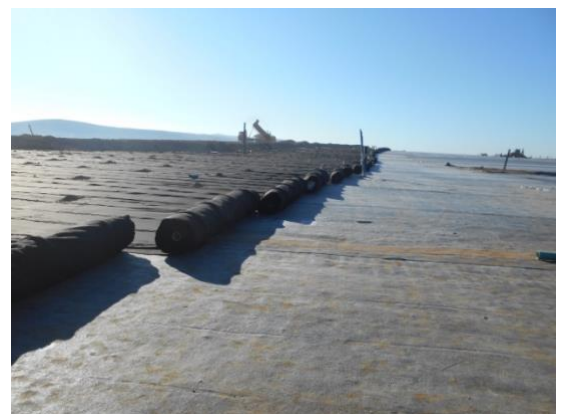
Roll -Up of DRAINTUBE FT on the GCL
