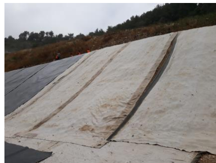
Installation of Géomembrane PEHD 2mm on GCL
