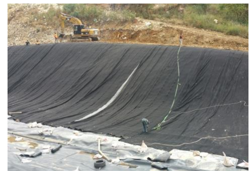
Installation of DRAINTUBE FT1 D16 on Geomembrane at slope
