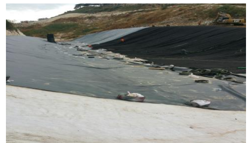
DRAINTUBE 400 FT1 D16 is installed above the Geomembrane
