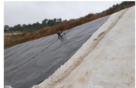
Installation and welding of Geomembrane PEHD 2 mm on GCL
