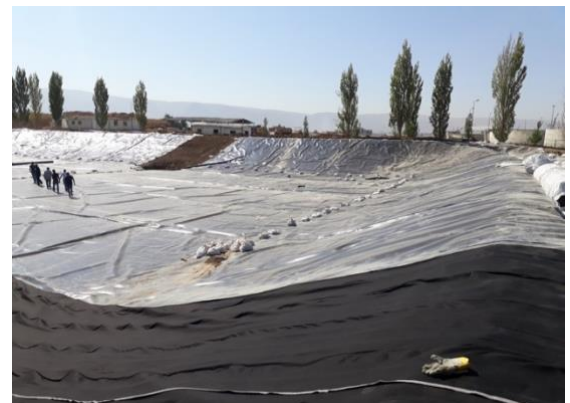
Installation of DRAINTUBE FT on geomembrane
