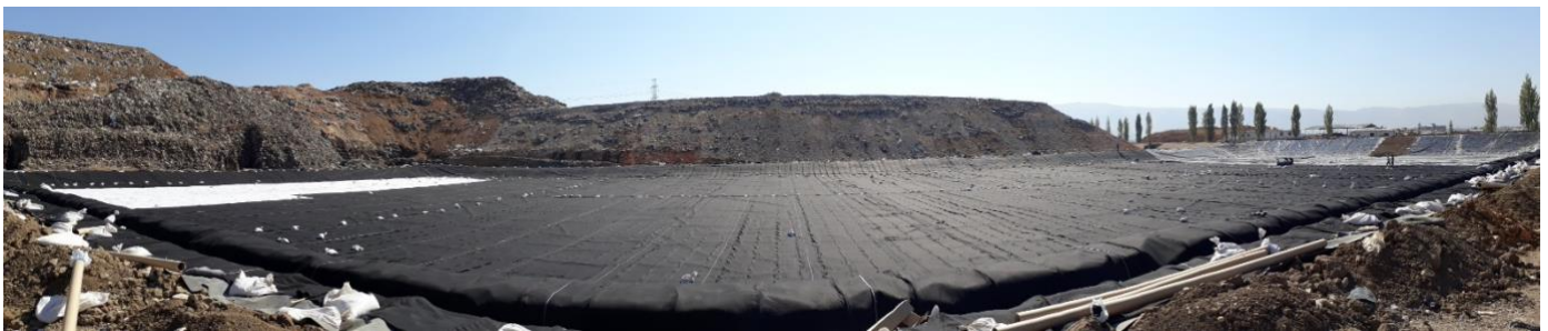
Unrolling of DRAINTUBE rolls on the Geomembrane
