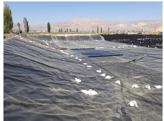
Installation of geomembrane (PEHD) on slopes and bottom of the cell
