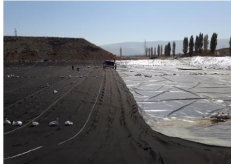
Unrolling of DRAINTUBE rolls on the Geomembrane
