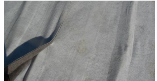
Overlap of roll lengths
