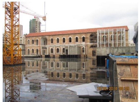
View of the site before the installation of COVERDRAIN FT
